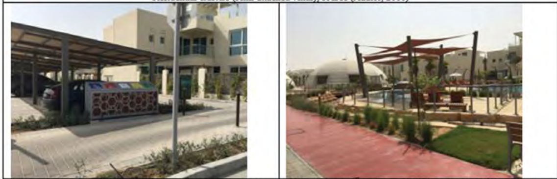
Parking shades covered with photovoltaic, and waste recycle bins are distributed among the city. Source (Author, 2016)
