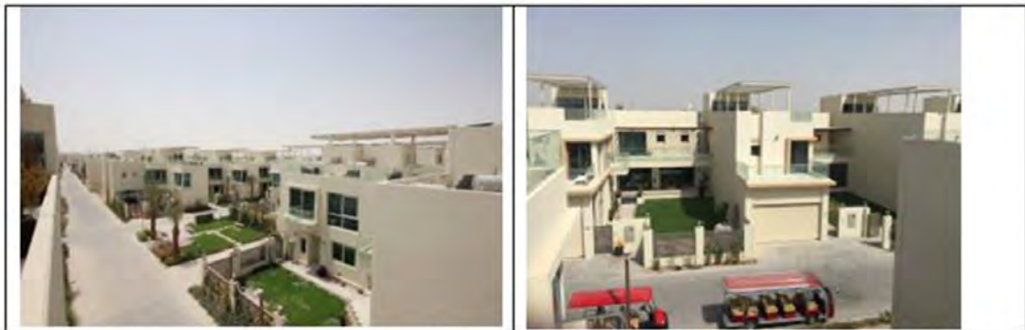
Residential clusters (semi-attached villas), source (Author, 2016)
