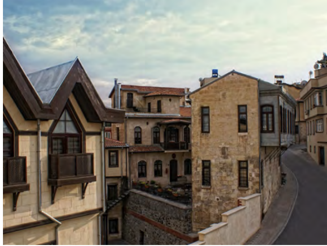
Figure 5. Current condition of Bey neighborhood (Bey Mahallesi, 2018).
