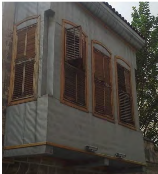
Figure 14. Wooden shutters (Taştan,2014)
