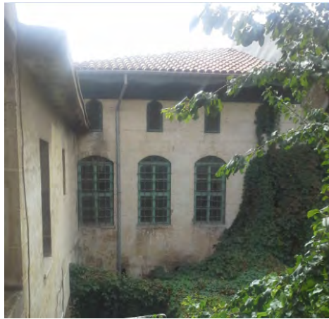
Figure 13. Bird Windows (Taştan,2014)
