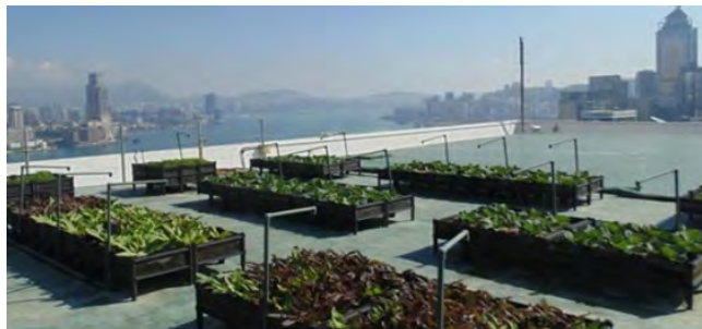
Figure 4. Farm built on the surface of the tower, “Bank of America” Hong Kong
