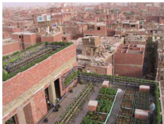
Figure 3. Greening Roof in unformed residential zone (Attia & Mahmoud, 2009)
