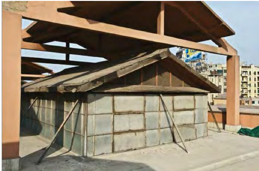
Figure 5. Roof modifications after 1967 war to protect it from air strikes (Photo by EQI report for reviving of the Egyptian museum in 2014)
