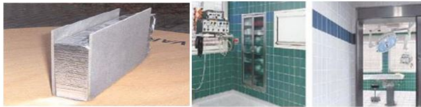
Figure 9. (VIPs) panels used in Operating theatre, Goslar,(Atwa, Al-Kattan, &Elwan, 2015, p. 3551-3564)
