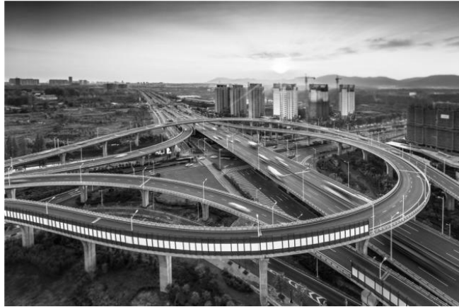
Figure 4 Three-dimensional traffic in Jiangbei New District
