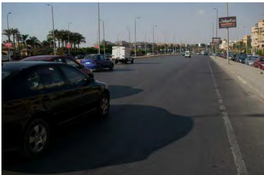
Fig. 29: 90th street before drain installment. (Source: the authors)
