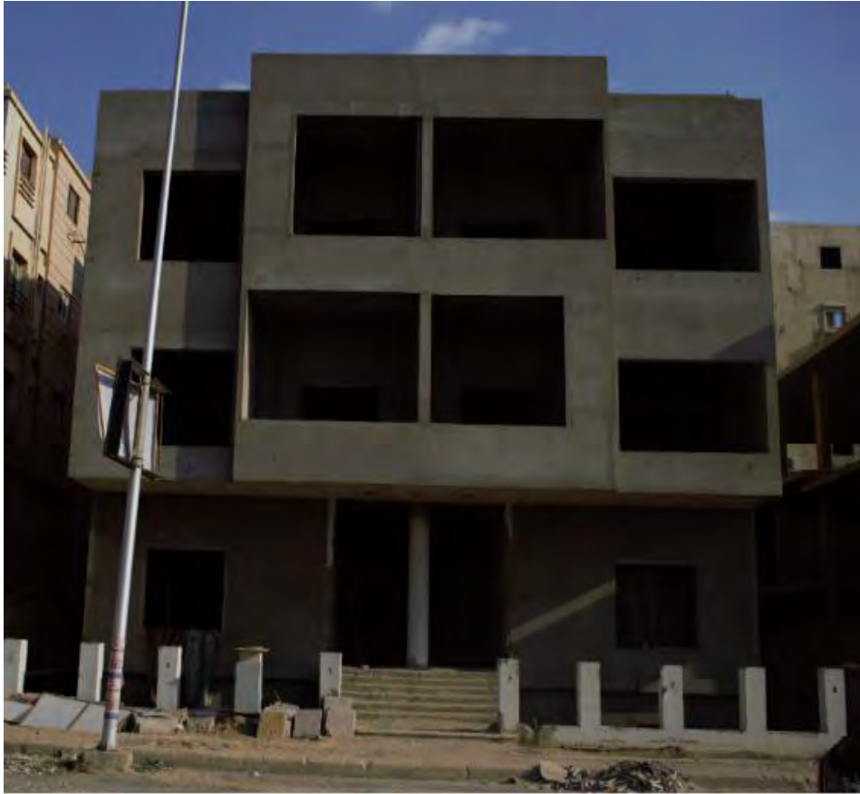
Fig 33: Building facades before vertical garden.
