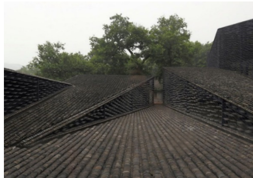
Figure 4. The outer wall is covered tiles and the roof
