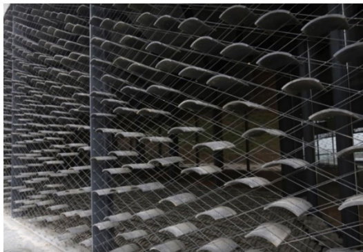
Figure 3. Applying old tiles for both the screen
