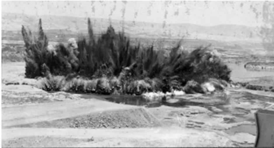
Figure 4: “Final major blast at The Dalles dam, removed 60,000 cubic yards of basalt, more than 20 tons of powder used.” 1956. OHS Research Lib, bb002863. [A black and white landscape photograph—A tall, mid-action dynamite blast stretches the length of the photograph, with clouds of dark smoke, dirt, and water extending skyward. In the foreground are gravel and sand bars, and portions of the Columbia River and low, smooth mountains are seen in the background.]
