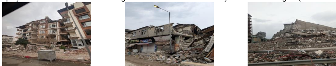
Figure 1: Damaged buildings after the 6 February 2023 Türkiye-Syria Earthquake
