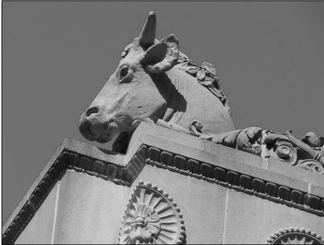
Figure 8. Architectural elements on Veterinary Hospital which is now Civil Engineering Building on Texas A&M Campus. Image courtesy of Rachel K. Turner.
