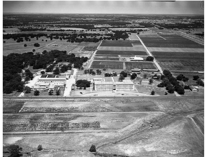
Figure 9. Completed Veterinary Medicine Complex in 1954 on University Drive, Cushing Memorial Library & Archives, Texas A&M University.
