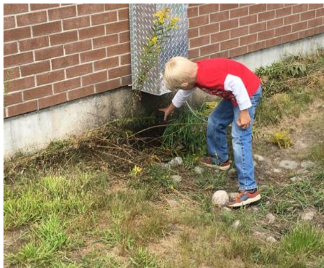
Figure 3. Drainage rain pipe
