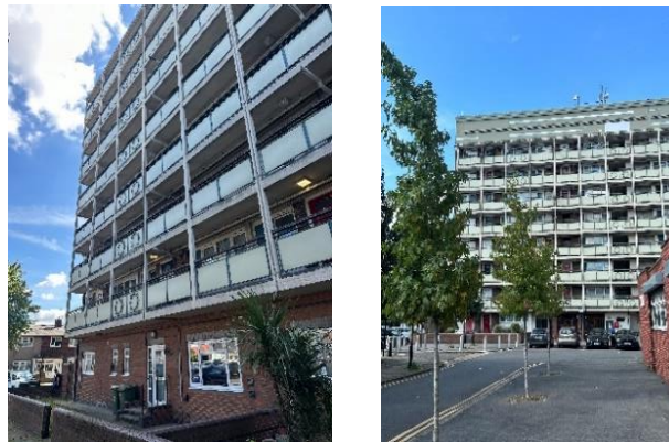
Figure 2: Case Study Buildings (Source: The authors)
