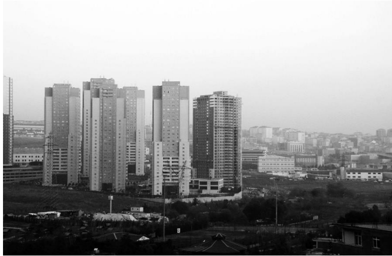
Figure 3: Rapid and uncontrolled urban growth in Istanbul: Urban housing (Özdamar, 2009)
