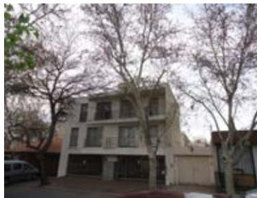
Figure 16. Views of the facade in autumn-winter season.
