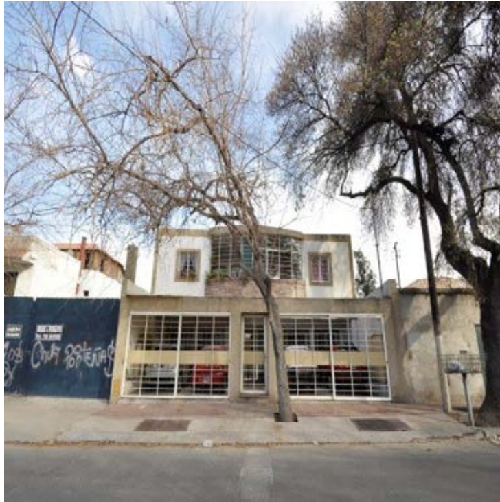
Figure 23. Frontal photograph of the facade.
