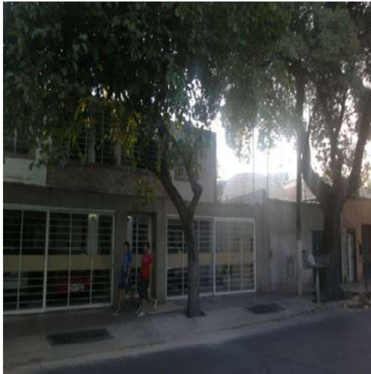
Figure 26. Frontal Photographs of the facade.
