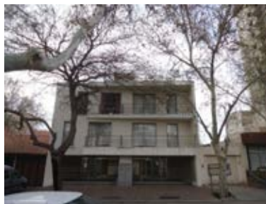
Figure 17. Views of the facade in autumn-winter season.
