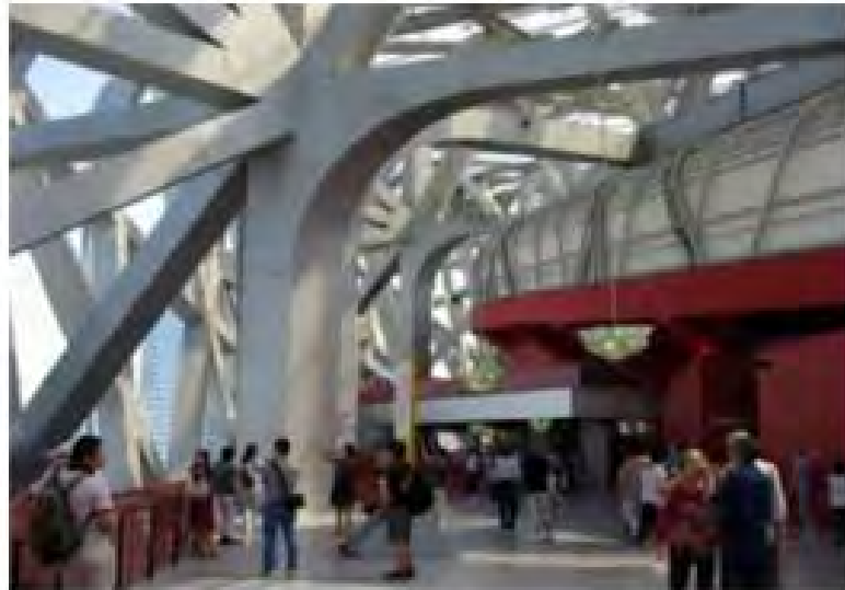
Figure 12. Bird'sNest Stadium n China, exterior.
