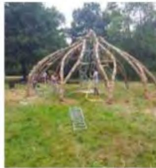
Figure 11. Structure after completion ("Turn Over a New Leaf", 2013)
