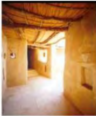
Figure 4. Roofing by Palm Rachis Adrere Amellal Eco-Lodge (Alamuddin, 2001)
