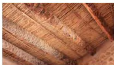
Figure 3. Palm Trunk Beams used for traditional roofing in Sinai (Ibrahim, 2010)
