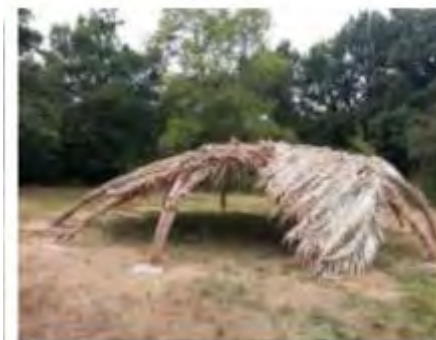
Figure 12. Deformation after sheathing ("Turn Over a New Leaf", 2013)
