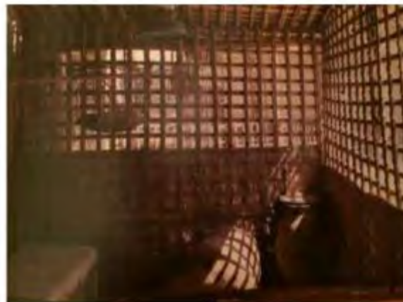
Figure 6. Date Palm Rachis walls and roofs in Arish House (Piesik, 2012)
