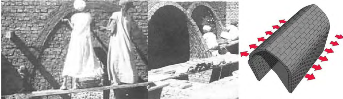
Figure 6. Depicts the roofing methods using the vaults
