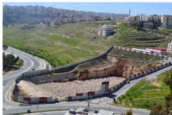
Figure 18. Sanaya Amman (Limitless towers) hole post filling it with sand and gravel. Source: Project: Manifesto, Holes on hold competition (2011)
