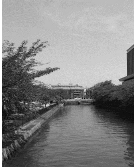
Figure 7. Lake Biwa Canal, Okazaki district Source: Taken by the author, 2015
