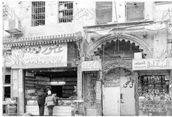
Figure 3. The façade of Wikālīṭ al-'Anbariyin . (Source: Al-Ahram online article, 2016 http://www.ahram.org/NewsQ/565296.aspx )
