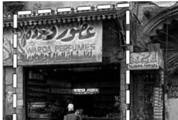
Figure 17. The white dashed rectangle indicates a shop that has its sign, before Wikāliī al-'Anbariyin demolition. Source: Al-Ahram online article, 2016
