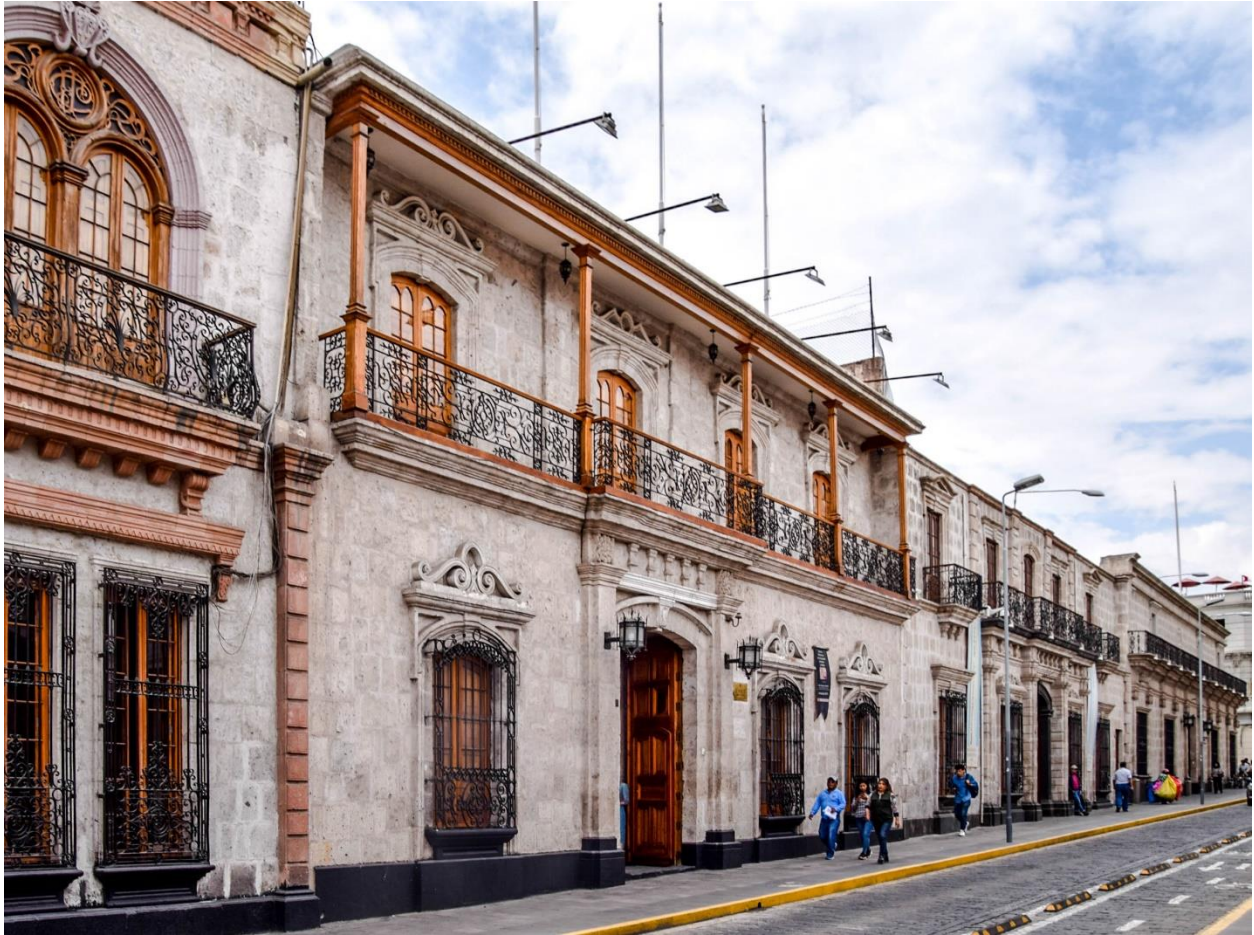
Figure 2. Façade of the building (Zeballos, 2019)
