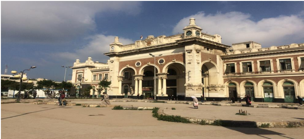
Figure 5: Egypt Railway Station Building - Alexandria (Part musings, 2015)
