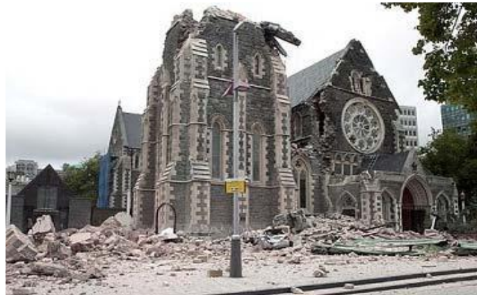
Figure 7: Christchurch Cathedral after the Earthquakes in 2011 (Telegraph 2011)
