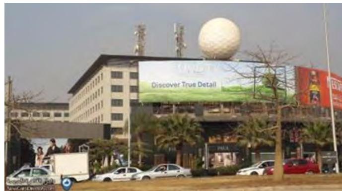
Figure 7. Downtown Mall Media Façade
