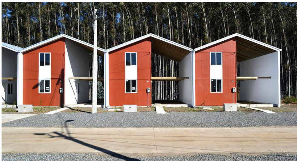
Figure 5: Elemental's Villa Verde project, Chile, with additional infrastructure over the incomplete half of the house. Archdaily, 2016.
