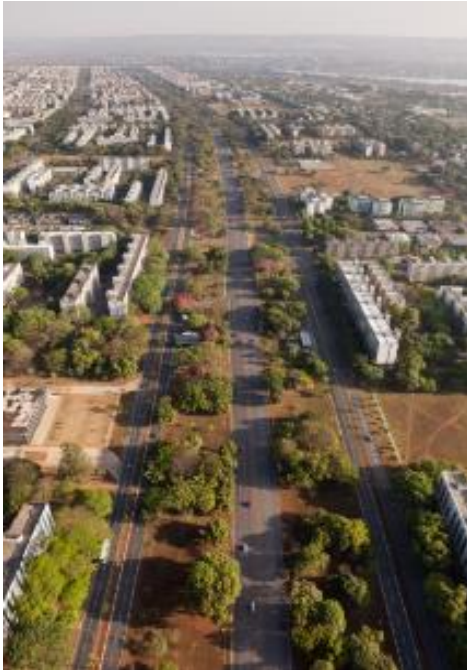
Figure 3 (right): Entrequadra 309/310 North. Between two Superquadras, this area is perceived as an empty area. Under the red polygon, there is a church, one of the common uses for this space. The highlighted area has 1.7 hectares approximately. (Base images extracted from Google Earth, 2021.)
