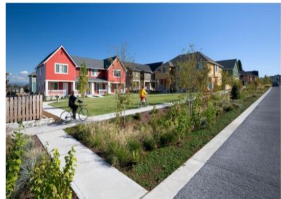
Figure 10: Swales in Seattle High Point.
