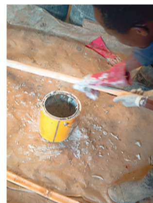
Fig. 2. Coating bamboo bars using Sikadur 32.
