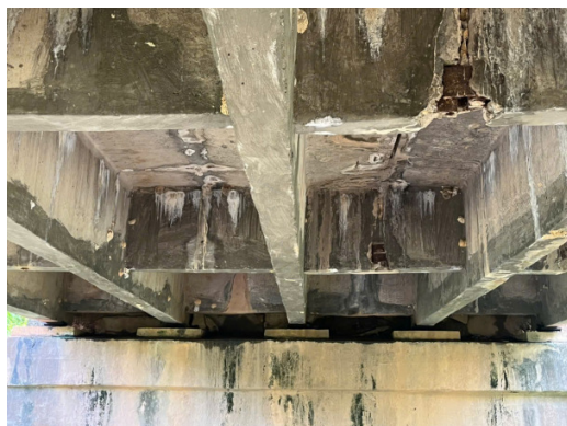
Fig. 1. Typical damage to simple span reinforced concrete bridges: (a) damaged bridge deck, (b) damaged bridge underside.
