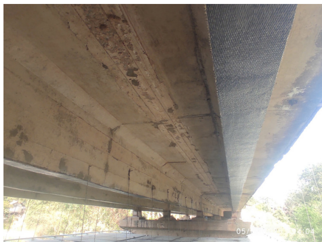
Fig. 10. Beam after application of carbon fiber reinforcement.
