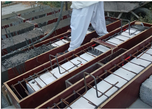
Fig. 5. Specimen preparation and casting.
