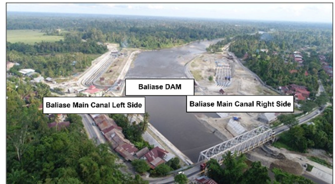
Fig. 2. Baliase Dam situation photo.
