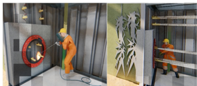
Fig. 4. The Injection process at the entrance hole in the starting pit area.
