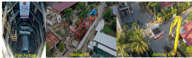
Fig. 2. Realization jacking pipe process.
