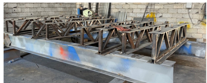
Fig. 6. Final manufacturing stage of DCTG and SCTG.
