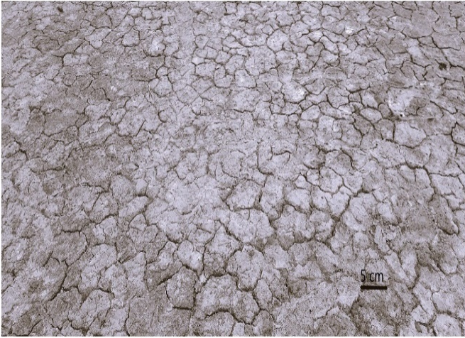
Fig. 1. Network of desiccation cracks in fine-grained soil.
