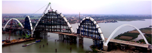
Fig. 6. Construction of deck and arches.
