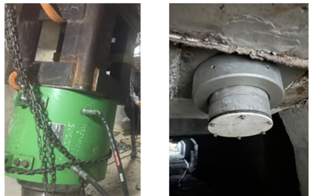
Fig. 7. Controlling the tension force in cables by pressure and elongation gauges.
