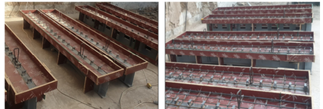
Fig. 15. Molds and bar reinforcement of specimens.
