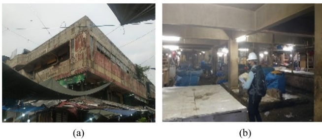
Fig. 1. External (a) and internal (b) view of the Merdeka Market building.
