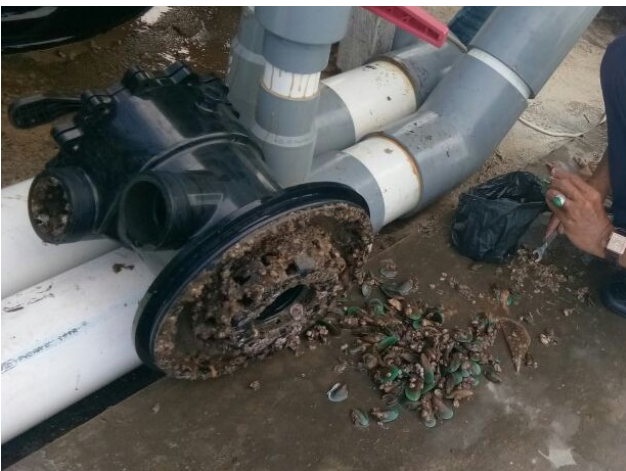
Fig. 7. The mouth of the sand filter is covered by green shells.
