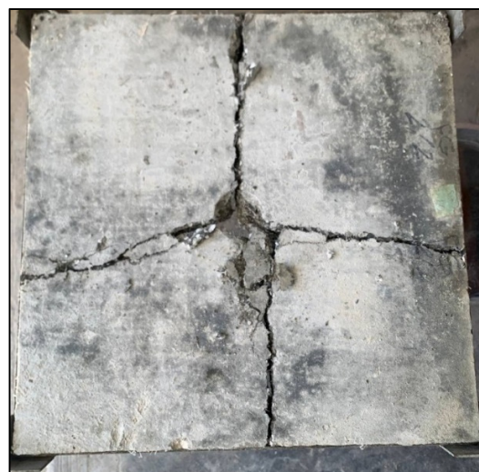
Fig. 3. The failure crack of one of the specimens.
