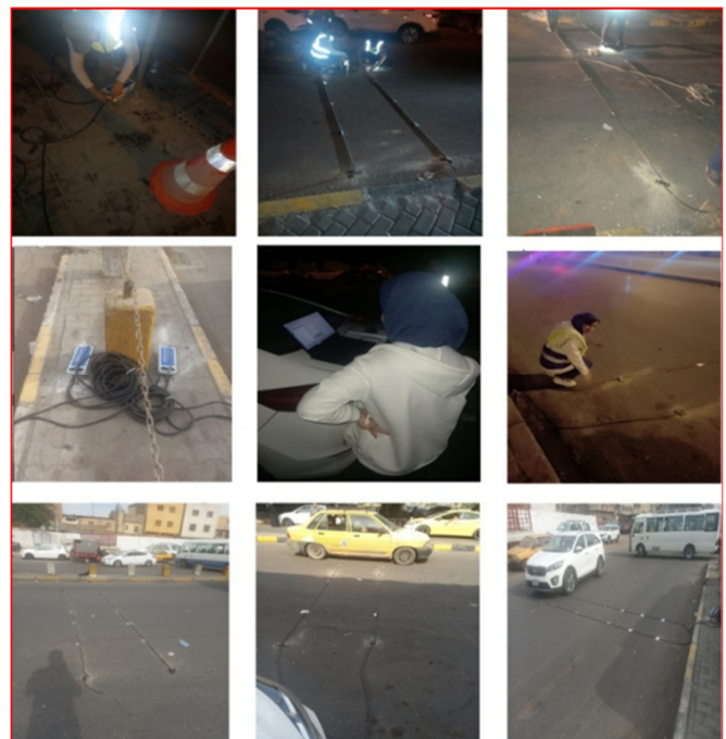
Fig. 2. Data collection using pneumatic tubes in the study area.
