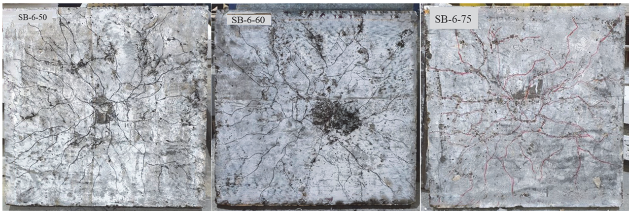
Figure 12: Crack patterns in 60 mm void bubble slabs after CFRP rehabilitation and re-testing to failure: (a) SB-6-50, (b) SB-6-60, (c) SB-6-75.
