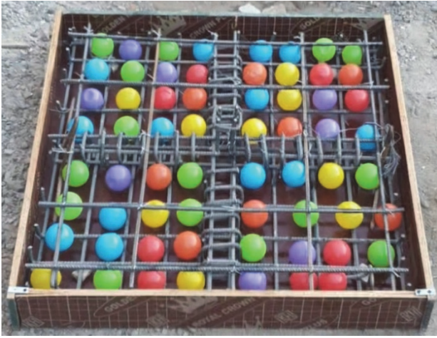
Figure 3: Casting of slabs.
