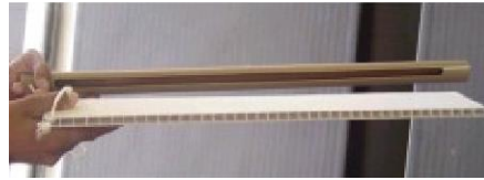
Fig. 2(b) Installation of PVC-B pipes with slots at the ends of the plates [11]
