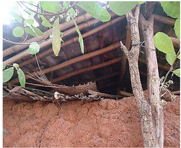
Fig.5 & 6: Falling old building and load bearing free wall showing fork wood carrying the roof. Photo: Okoroafor.
