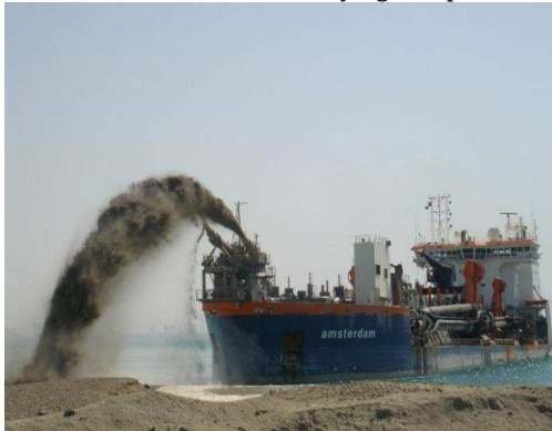
a) Hydraulic dredging system
