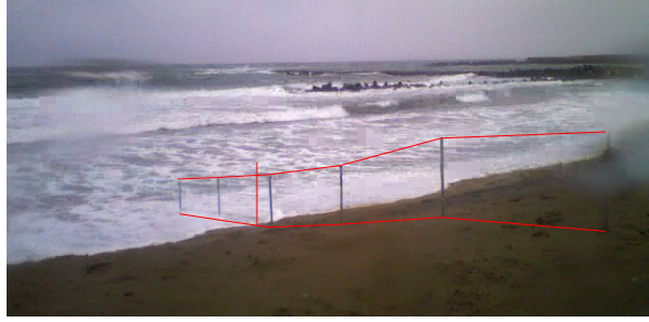
Figure 5 Photo of wave runup on the foreshore taken on 2 March, 2021.
