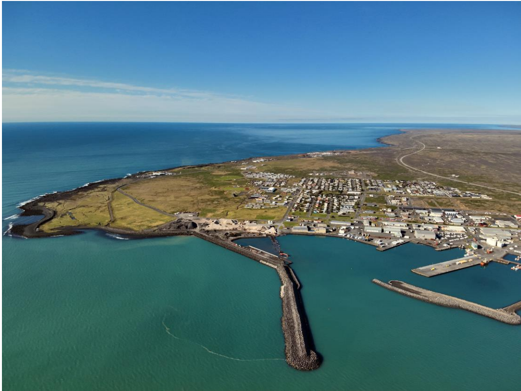
Figure 2. The port of Thorlakshofn after the 250 m elongation of the breakwater in August 2024 (photo Pall Marvin Jonsson).
