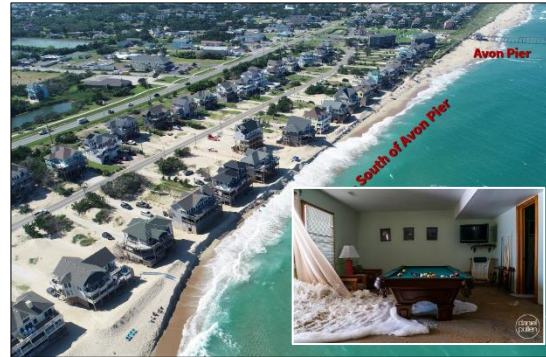
Figure 6. Aerial photo taken on 15 July 2020 looking north, showing the highly eroded section of Avon south of the pier. The ground photo was taken by Daniel Pullen on 20 September 2020 during Hurricane Teddy . NC Highway 12 was closed for 5 consecutive days due to overwash caused by ocean swell generated by Teddy (USACE 2021b).
