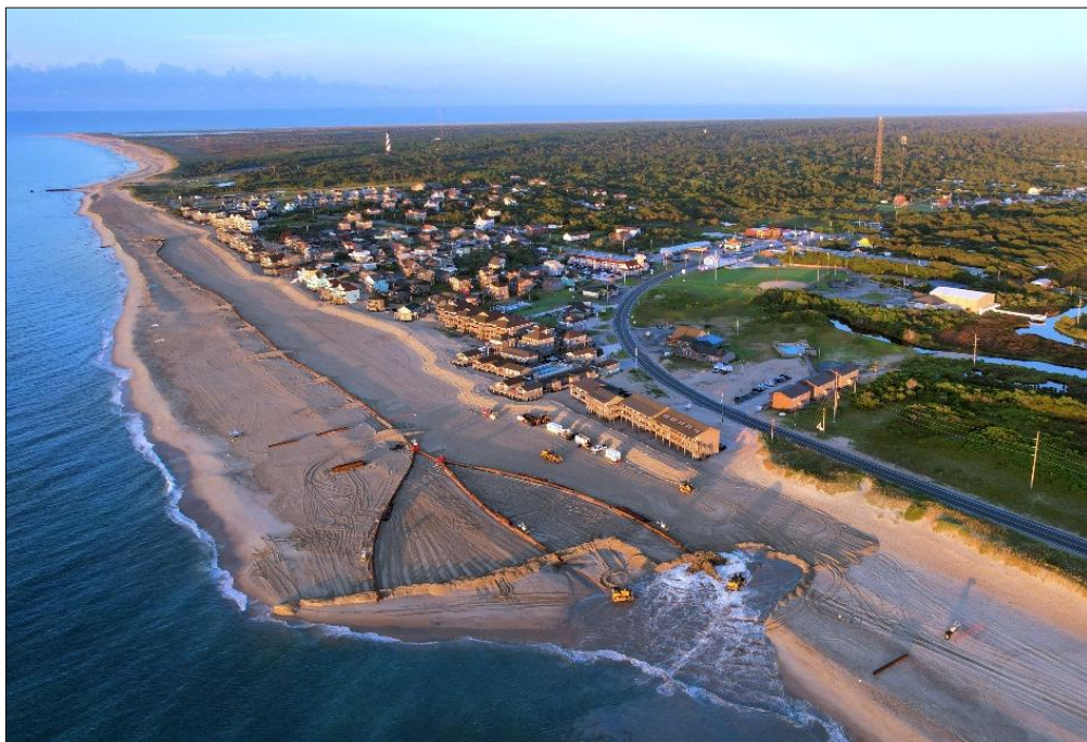
Figure 9. Oblique aerial images on 5 August 2022 during construction of the 2022 Buxton beach renourishment project.
