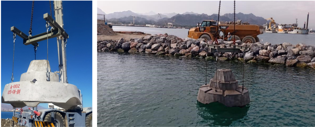
Figure 3. ACCROBERM™ I units installed on a project site in 2019
