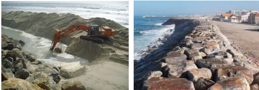
Figure 1. Reinforced coastal revetments: left) works deepening the foundation of a longitudinal revetment at Vagueira, Portugal; right) increased crest level of a longitudinal revetment at Esmoriz, Portugal.
